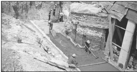
Roman Fort Work in Progress
