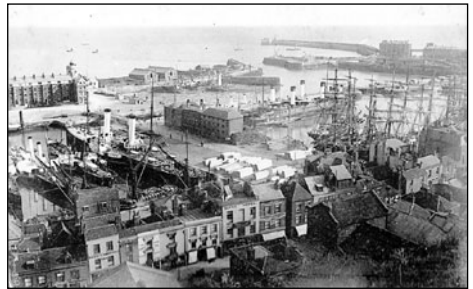
Western Dover Harbour Docks
