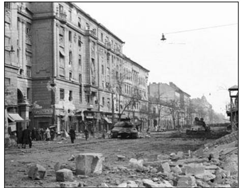
Rubble after the end of the fighting in Budapest's 8th District 1956
