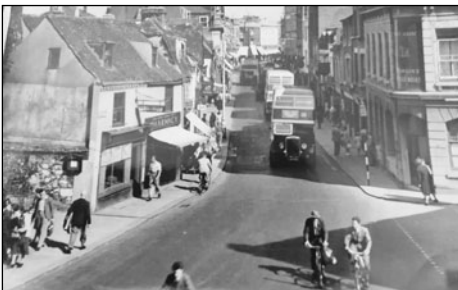
Biggin Street Before Widening
