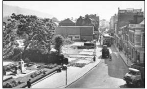
Biggin Street After Widening
