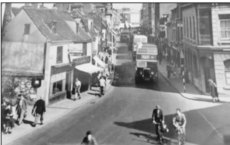
Biggin Street Before Widening
