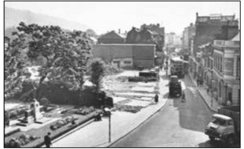
Biggin Street After Widening
