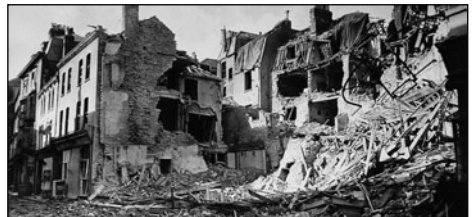
WWII Shell Damage Snargate Street at Five Post Lane
