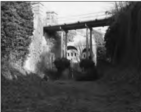
Fort Burgoyne Bridge
