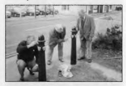
During 1993 Environment Week restoration of Dover's 'leopard bollards' by the Society began in various parts of the town. St. Mary's School pupils assisted a team of four in removing old paint down to the bare metal, priming and painting the bollards black and finally gilding the leopards' heads and bollard tops. After sessions every Saturday from March to May the job was finished and Joe Harman's dream realised. The annual
