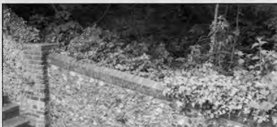
Effingham Steps after final clearance
