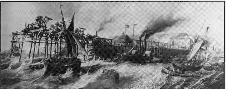
Construction of the Admiralty Pier
