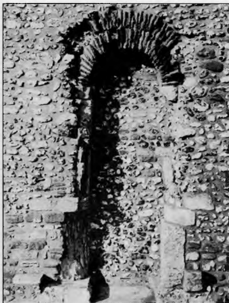
The old Saxon south door as it is today after being excavated and exposed to the elements since the 1860's.
