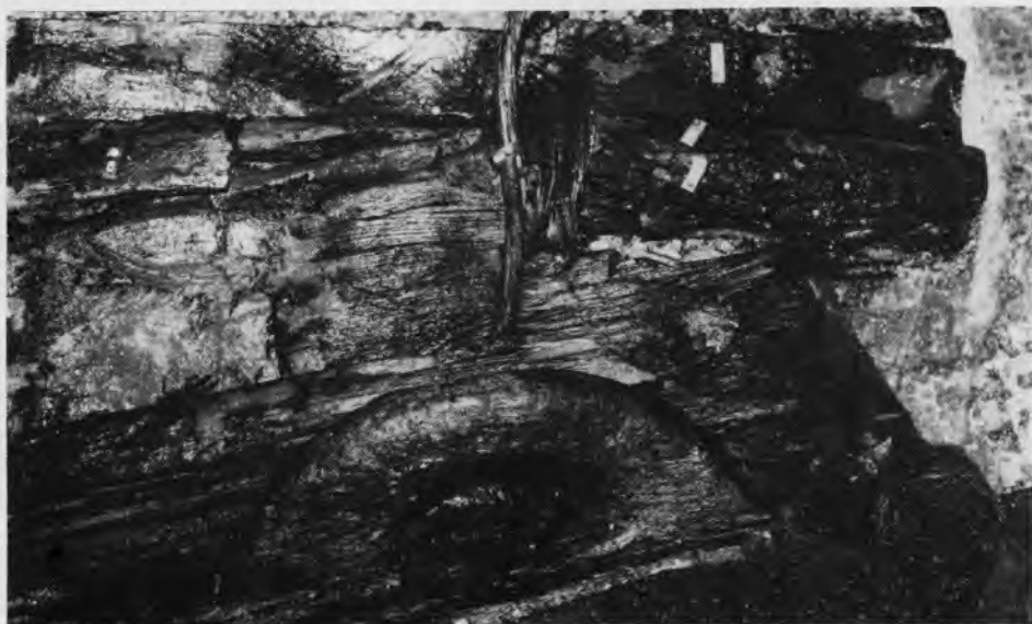
PLATE II: Detail of the boat's construction, showing a carved side cleat (uncertain purpose) and a twisted yew wood with which held the individual planks in place.
