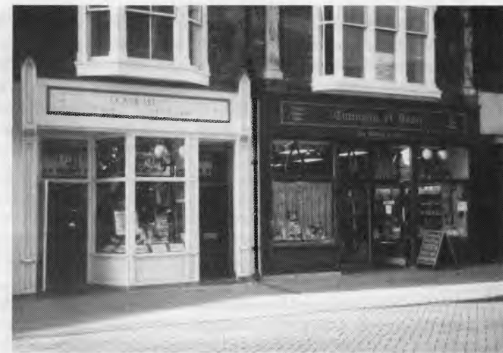
THE RESTORED SHOPS IN CANNON STREET
