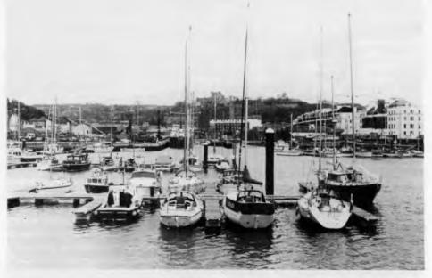
Dover Harbour Board has recently installed 67 new pontoons in the Wellington dock. This brings the total number available to 104. Each berth is equipped with running water and a 13 amp electricity supply. The pontoons were designed, constructed and installed by Simmonds Marine (Projects) Ltd.
